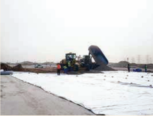
ALYAF SALT BARRIER being installed at the Orbital Highway Project at Qatar
